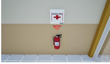
Figure 9 Placement of Fire Extinguisher & First Aid Kit at Faskampen Laboratory
