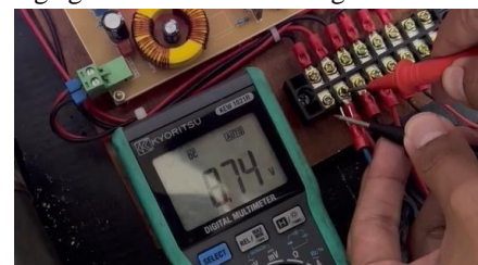
Figure 4 No-load Generator Measurement
