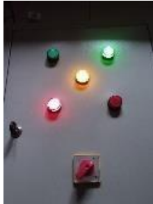
Figure 4 Testing the Load Switching Monitoring System
