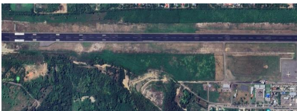
Figure 4. 3 Mobilization path and material disposal location (Source: Google Earth, accessed May 14, 2024)
