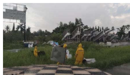
Figure 3.1 The affected GSE Storage areas
