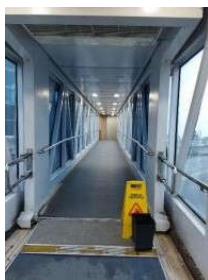
Figure 1 The condition of the garbarata
