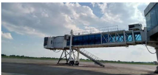
Figure 3.2 Broken Garbarata at Parking Stand 8 Source: Author (2023)
