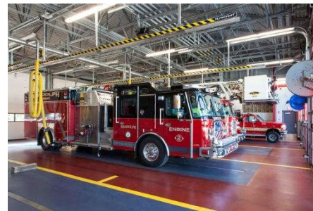
Figure 6. Vehicle Housing with Epoxy Layer
