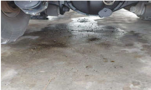
Figure 2. Floor Surface Exposed to Oil Spills
