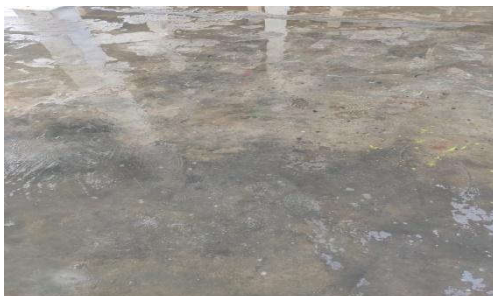
Figure 4. Post-Cleaning Floor Condition
