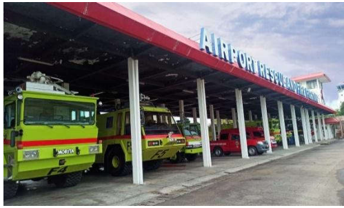
Figure 1. ARFF Vehicle Garage, Hang Nadim Batam International Airport.
