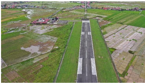
Gambar 1 View Drone Runway Strip Eksisting dan Drainase Eksisting Sumber: Penulis, 2025
