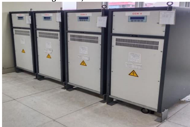
Gambar 1. Constant Current Regulator
