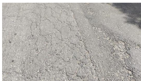
Figure 2. Aligator Cracking
