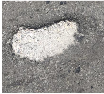
Figure 3. Patholes Source : Reseachar Data
